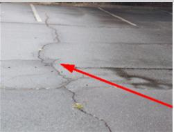
The driveway is cracked and displaced. The raised section of the driveway has created a path for water penetration under the slab and a trip or fall hazard. A licensed general contractor should be consulted for further evaluation and repair.
