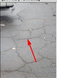
The driveway is cracked and displaced. The raised section of the driveway has created a path for water penetration under the slab and a trip or fall hazard. A licensed general contractor should be consulted for further evaluation and repair.
