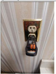
The building was built before GFCI circuits were required to protect all electrical receptacles located outside or within six feet of water. GFCI circuits add an important safety feature to electrical systems. The buyer should consider upgrading the electrical system to include GFCI protection.
