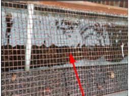
Standing water was noted in the gutter trays in several locations. This indicates that the gutters are not draining and could indicate improper tray slope, a clogged exits, or downspout extension. Direct drainage to the foundation and cladding from the gutter system can result in water penetration into the foundation area and foundation deterioration. A licensed general contractor should be consulted for a complete evaluation of the gutter system to reduce overflow and to make necessary repairs.
