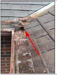
Evidence of debris in the valley impeding gutters from working properly. Direct drainage to the foundation and cladding from the gutter system can result in water penetration into the foundation area and foundation deterioration. A licensed general contractor should be consulted for a complete evaluation of the gutter system to reduce overflow and to make necessary repairs.
