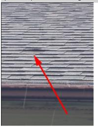
Exposed nails have displaced shingles over the roof surface. Displaced shingles could indicate an underlying problem with the shingles installation or attic conditions. A licensed roofing contractor should be consulted for a complete evaluation and to make necessary repairs to ensure the weathertightness of the roof covering system.
