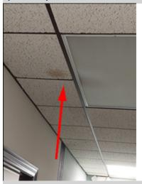
From the attic, the wood framing components located in an interior room are discolored. The framing, insulation, and ceiling show evidence of a history of a leak. A licensed general contractor should be consulted for further evaluation and repair to determine the source of the leak and extent of the damage to ensure the stability of the home and prevent additional damage.
