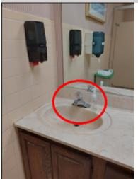
The faucet in the women's bathroom is not connected properly and loose. This could leak to leaking water pipes. A qualified technician should be consulted for further evaluation.
