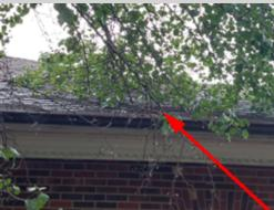
The shingles for the building are covered with a heavy build-up of leaves/pine needles/debris. This limited the inspection of the roof surface. Debris on the roof surface can trap moisture allowing water and debris to travel under the shingle tabs resulting in material failure and leaks. A roofing contractor should be consulted to remove the debris and inspect the shingles/adjacent component for evidence of damage and make necessary repairs.
