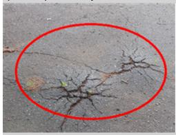
The driveway is cracked and displaced. The raised section of the driveway has created a path for water penetration under the slab and a trip or fall hazard.
