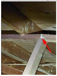
From the attic, the roof rafters were noted to be bowed or warped beyond what would be typically expected. The bowing could indicate an underlying problem with the rafter design, installation, or attic conditions. An engineer should be consulted for further evaluation to determine the significance of the concern and outline necessary repairs to ensure the stability of the structure.
