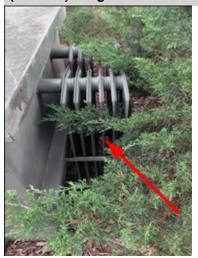
The vegetation around the transformer of the building is over grown and blocks the air circulation around the transformer. A landscaping company should be consulted to correct the over growth and the inspection should be completed prior to purchase.
