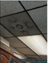
Ceiling diffuser for HVAC show signs of previous moisture in system. There is no obvious dripping at time of inspection. Further evaluation is recommended by qualified HVAC contractor to review.
