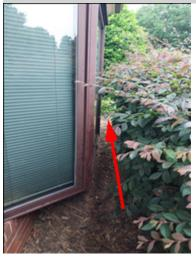
The vegetation around the perimeter of the building is over grown and blocks the air circulation around the building. The growth also limited the inspection access. A landscaping company should be consulted to correct the over growth and the inspection should be completed prior to purchase.
