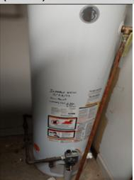
The water heating unit for this building is 9 years old. A water heating unit has a life expectancy of 10 to 12 years. The unit was noted to be operational and fair condition. The unit should be serviced annually and the TPRV inspected and or replaced every three years. The buyer should budget for replacement.
