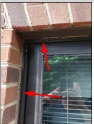
All windows in building need to be caulked and sealed to avoid water penetration. Water penetration will lead to rot and mold. A licensed general contractor should be consulted to determine the extent of the damage and make necessary repairs.
