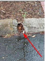
Drain is clogged with leaves and debris. A licensed general contractor should be consulted for a complete evaluation and to make necessary repairs.
