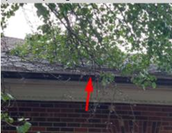
The vegetation/tree limbs around the perimeter of the building is over grown and blocks the air circulation around the building including the roof. The growth also limited the inspection access. A landscaping company should be consulted to correct the over growth and the inspection should be completed prior to purchase.
