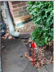
The gutter downspouts are not extended or piped correctly to direct roof drainage away from the foundation. Direct drainage to the foundation and cladding from the gutter system can result in water penetration into the foundation area and foundation deterioration. A licensed general contractor should be consulted for a complete evaluation and to make necessary repairs.
