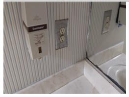
The building was built before GFCI circuits were required to protect all electrical receptacles located outside or within six feet of water. GFCI circuits add an important safety feature to electrical systems. The buyer should consider upgrading the electrical system to include GFCI protection.
