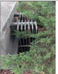
Transformer requires airflow around the exterior to keep it functioning as intended. According to label shrubs, trees etc. should be cleared 10 Ft around unit.
