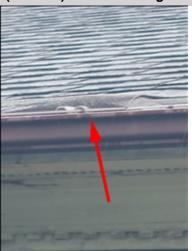
An installed condensate drain has shingles bunched up on eave. Further investigation is recommended by a licensed contractor.
