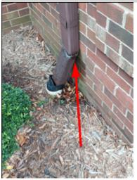
There are several gutter downspout that are damaged and working improperly. Direct drainage to the foundation and cladding from the gutter system can result in water penetration into the foundation area and foundation deterioration. A licensed general contractor should be consulted for a complete evaluation and to make necessary repairs.
