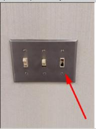
The switch for the light fixture is broken. Damaged switches could result in improper operation of fixtures and electrical hazards. A licensed electrical contractor should be consulted for further evaluation and to make necessary repairs.
