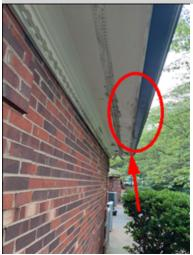
The gutter trays have been leaking at seams and corners. It is very important to keep gutter functioning properly to reduce direct drainage to the foundation and wall cladding systems. A licensed general contractor should be consulted a complete evaluation and to make necessary repairs.
