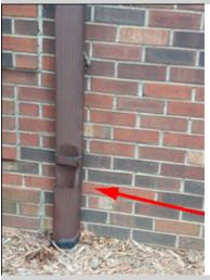
There are several gutter downspout that are damaged and working improperly. Direct drainage to the foundation and cladding from the gutter system can result in water penetration into the foundation area and foundation deterioration. A licensed general contractor should be consulted for a complete evaluation and to make necessary repairs.
