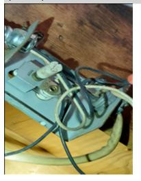
There is an open junction box located in the attic for fan control this a possible electrical shock hazard. Recommend a licensed electrical technician evaluate.
