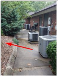
The grading around the package HVAC unit is directing drainage toward the unit and into the building. Direct water penetration into the slab is undesirable and should be corrected. A licensed general contractor should be consulted to make necessary repair to ensure correct lot drainage and that the foundation area will be dry and stable.
